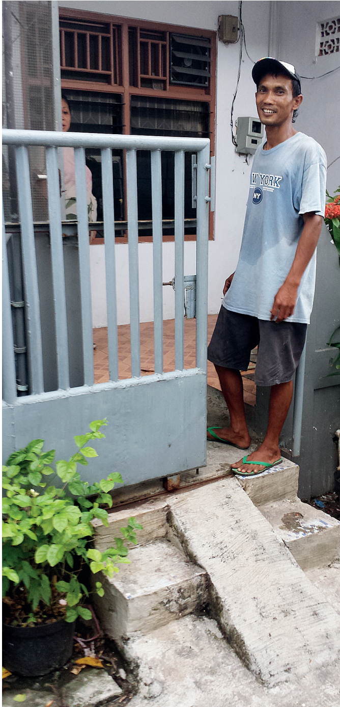
Above, residents of middle class neighborhood sometimes raise the first floor above street level.
