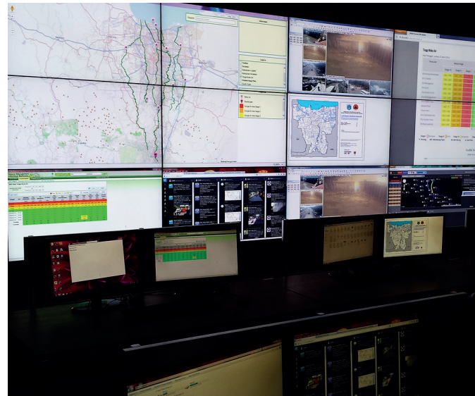
Pusdalops control center decision-making tools, including maps, real-time flood data, and live streaming camera pointed on the dam
